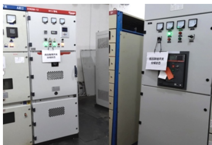
Modification of high and low voltage switch board room
